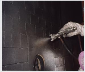
Coating refractory lining
