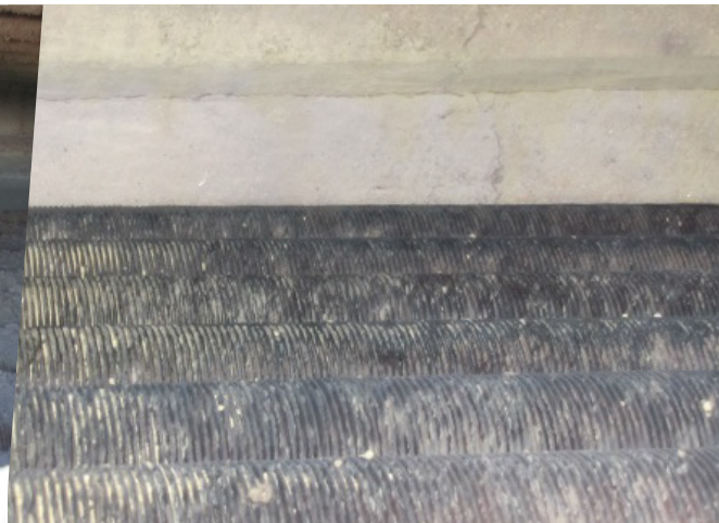
Hot convection section cleaning completed
