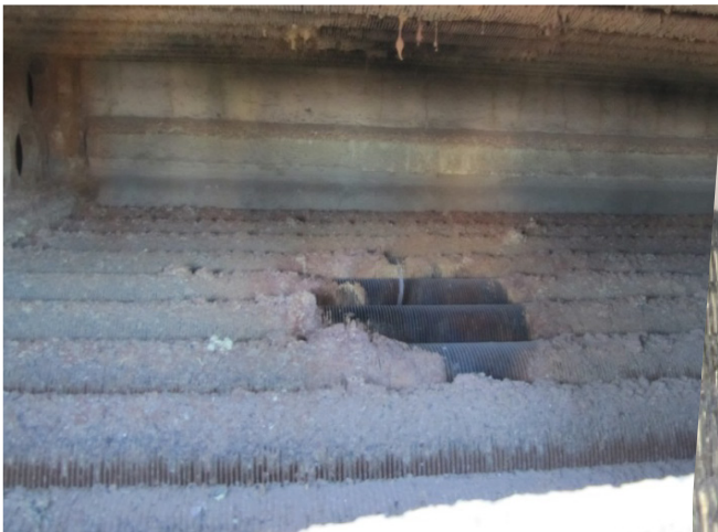
Hot convection section cleaning in action
