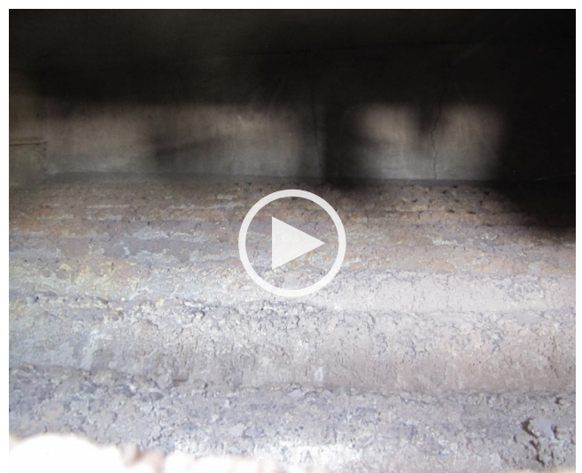
Convection section fouling, watch this application in action
