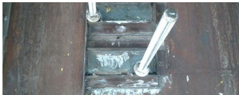
3. Finished application (exterior)
