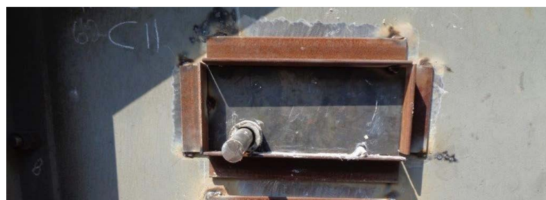
3. Tube stabilizers installed awaiting final welding (outer view)
